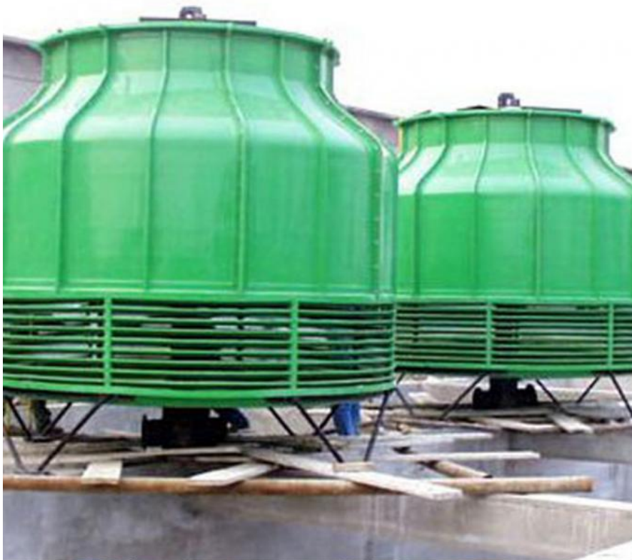
Round counter flow cooling tower---wind direction ↑ from Tower bottom air intake
