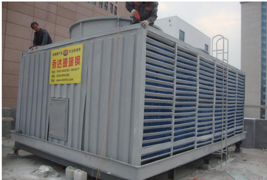
Square cross flow cooling tower ----wind direction ← from the standing side of the tower
