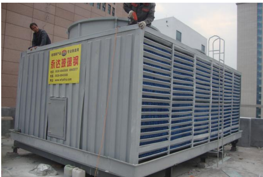
Square cross flow cooling tower ----wind direction
